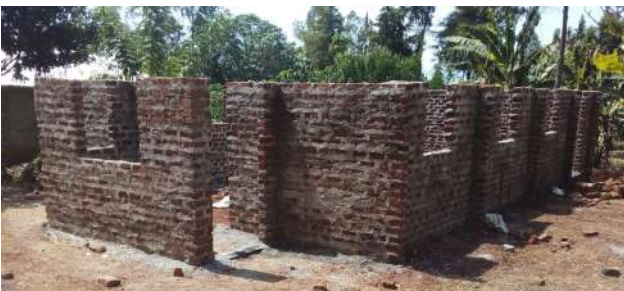
GOA Nyasita in Nyanza is in its first phase of building
